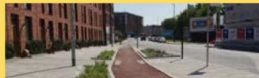
Figure 21. Example of a SUDS segregated cycle track
